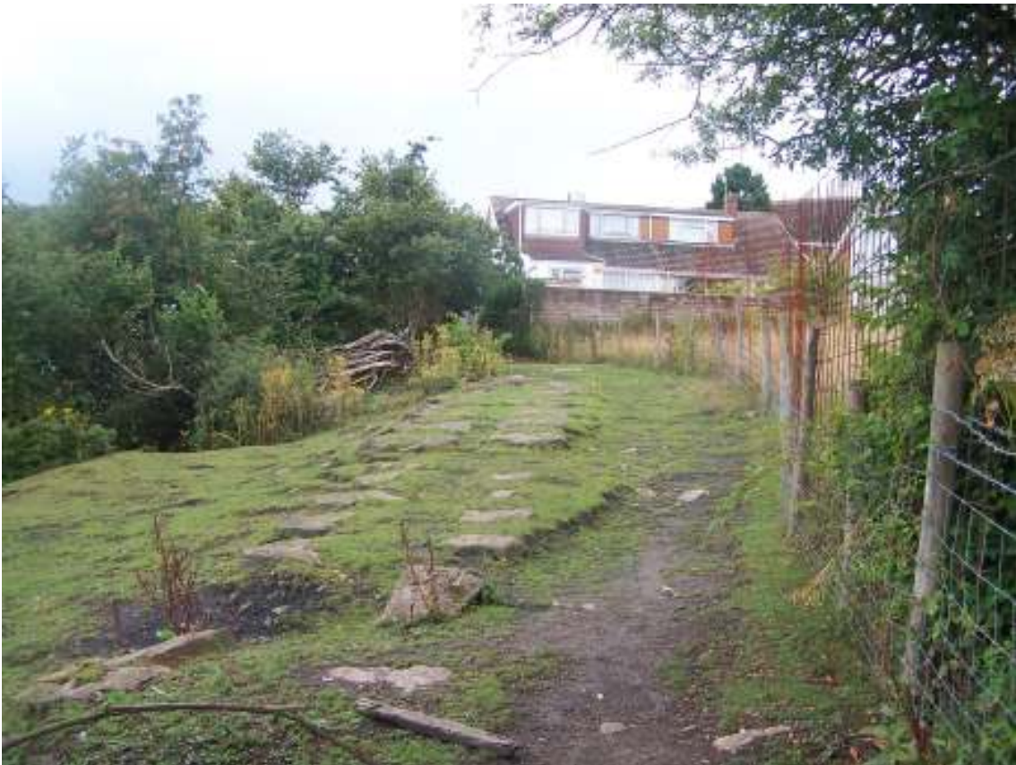
Stone blocks on a former plateway to ironstone quarries, Heolgerrig, West Merthyr; the pressure of urban development on the monument is clear.
